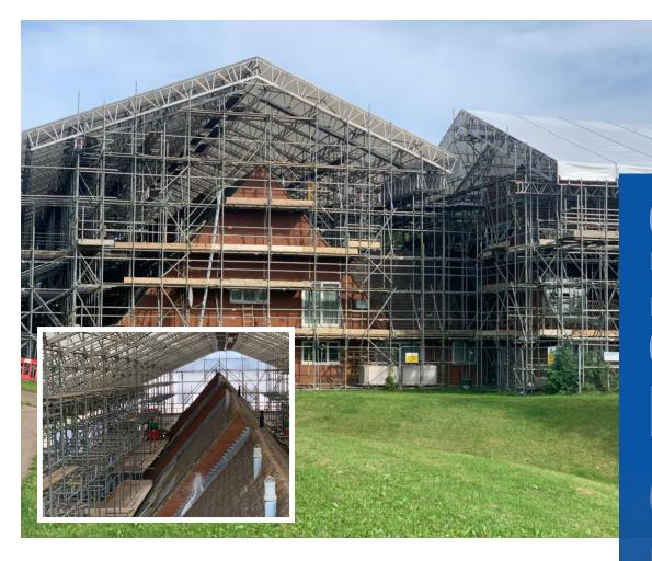
Faced with providing two temporary roofs over a steeply pitched roof, High Standards Scaffolding of Hemel Hempstead found the perfect solution: Their inhouse design team integrated the company's own stock of tube and fittings to support the roof with two Haki temporary roofs supplied by UK System Scaffold Hire.
