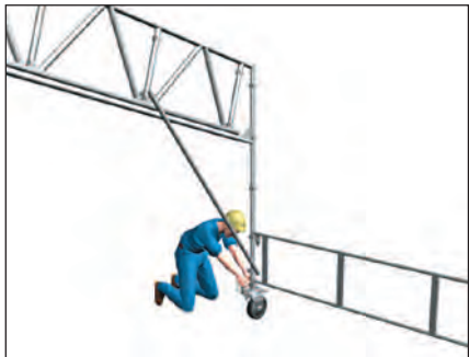
Figure 15 Adjust Wheel/base Jack if ground level requires.
