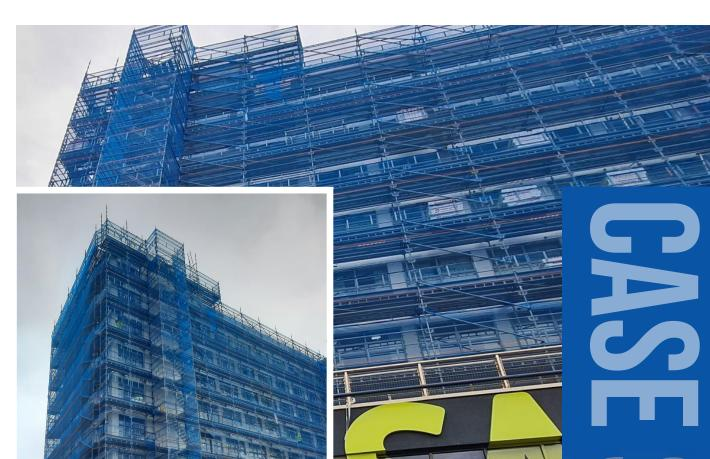
By designing scaffold with a 3-metre lift, UKSSH and XL Scaffolding made the removal and replacement of cladding quick and easy at the Ice House - an iconic building in the centre of Nottingham.
