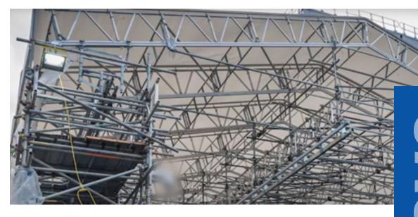
Working closely with Creator Scaffold Design, UKSSH supplied a Haki Temporary Roof that enabled a redundant sixty-yearold settling tank at Sellafield to be cleared of radioactive sludge and then be resealed in record time.
