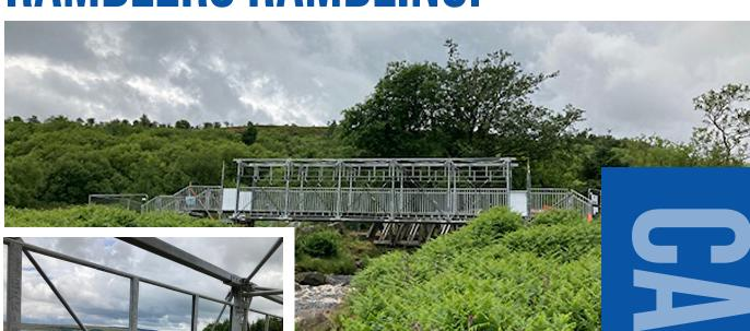
Many of UKSSH's projects using the Haki **Bridge System (HBS) and Public Access** Staircases are notable for the challenges that they overcome, be it restricted access to site, short possessions or the span of the bridge. However, the simplicity of the HBS makes it the ideal solution even for relatively "simple" projects, as SYS (Scaffolding Contractors) Ltd and UKSSH proved at Grimwith Reservoir.
