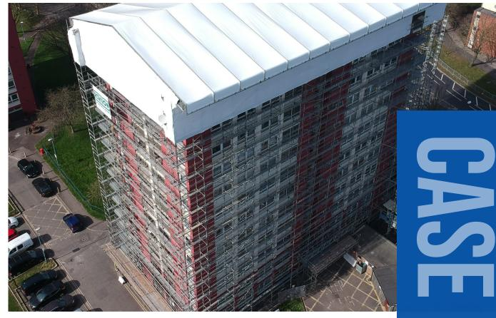
Installing a Haki temporary roof on the top of a 12-storey block of flats is one of the more dramatic ways to demonstrate the many benefits of Haki System Scaffold, but the project at Baynton House in Bristol proved to be the perfect platform for a collaboration between Ashton Scaffolding and UK System Scaffold Hire.
