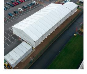
The HAKITEC Temporary Building provided the ideal solution: There was no need for civil engineering base works and the product is even designed to quickly overcome problems such as uneven or sloping sites.
