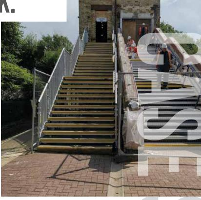
The temporary stairs mimicked the permanent stairway thus fitting within the confines of the station and maintaining station operations throughout and the stair landings where covered with non-slip GRP."
